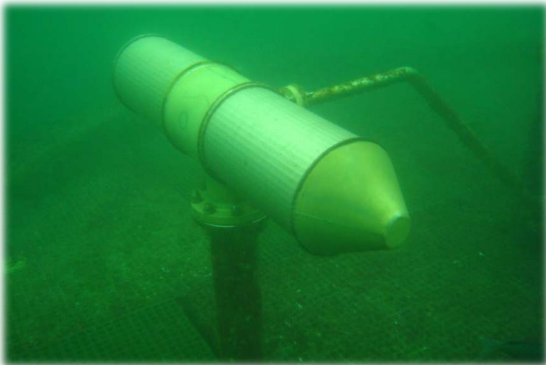
Figure 10-5: Potential Wedge-Wire Intake Configuration
