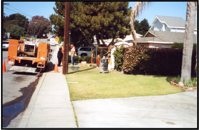
Fig. 6-5. PUMP STATION NO. 6 SITE In Palm Avenue East of California Street
