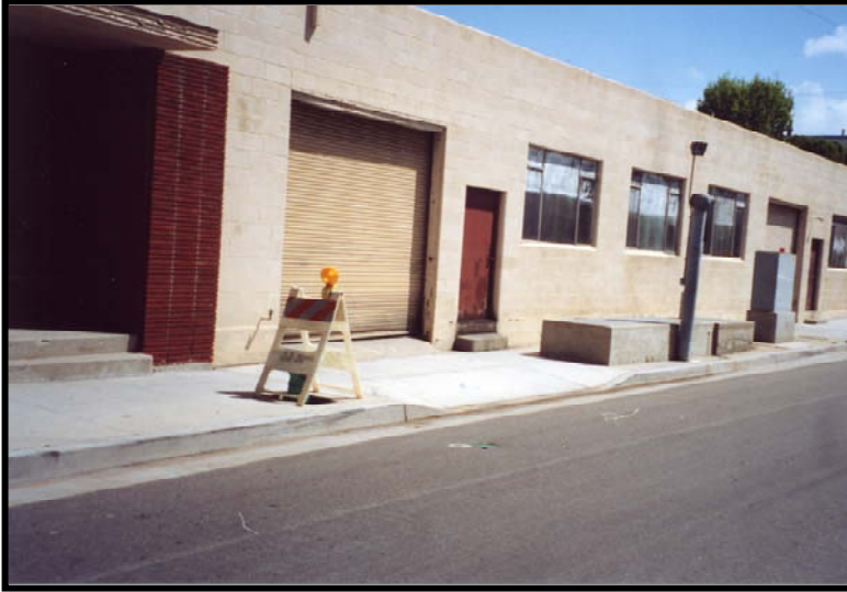
Fig. 6-3. PUMP STATION NO. 2 SITE In Franklin Avenue West of Arena Street
