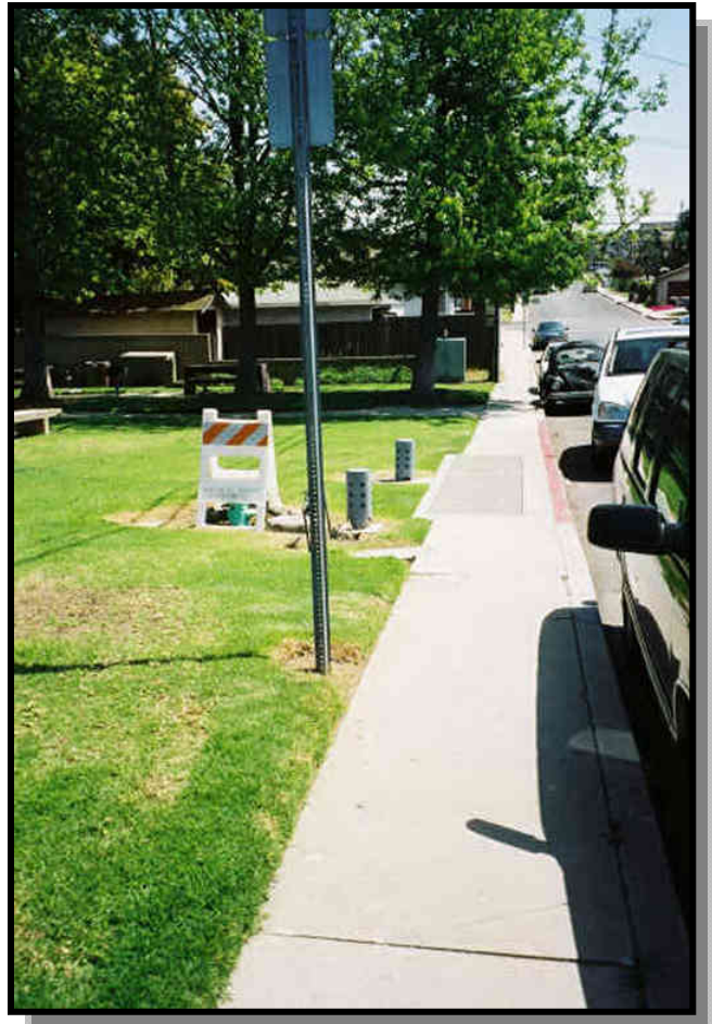
Fig. 6-1. PUMP STATION NO. 1 SITE In Acacia Avenue West of Loma Vista Street
