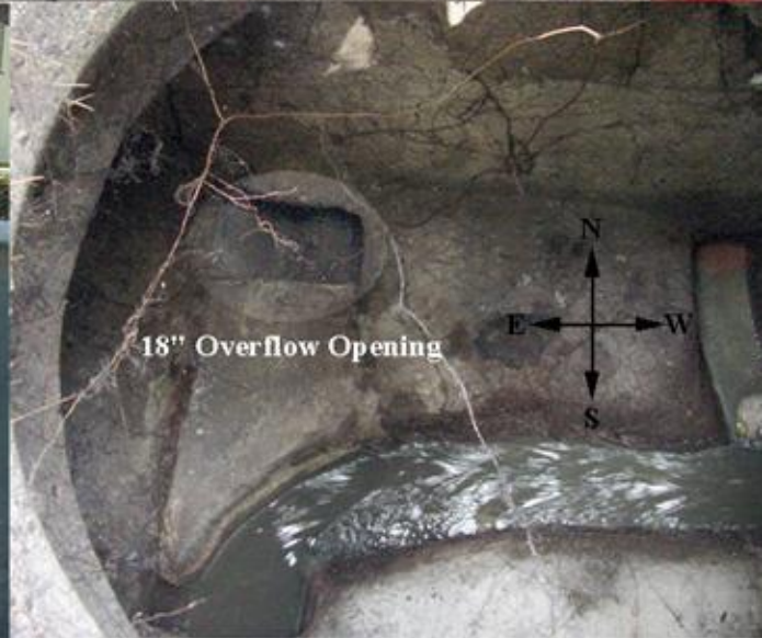
View inside 18" Overflow Manhole
