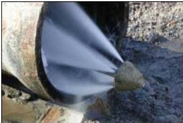
Figure 3. Jetting an exposed pipe.
