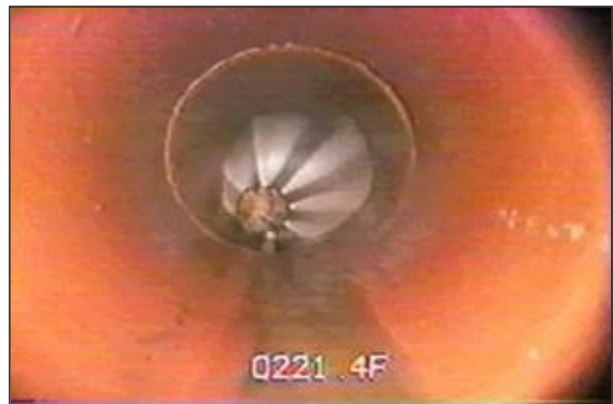
Figure 4. Jetting a sewer main.
