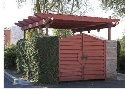
Trash enclosures with architectural screening elements
