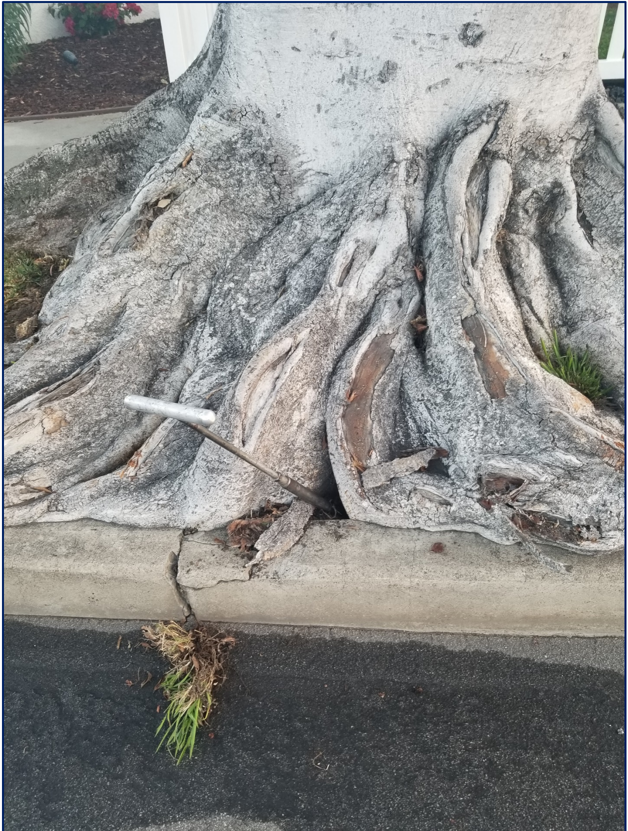
Image 12. Sowing the cavity in the buttress, the probe was inserted 10-inches.
