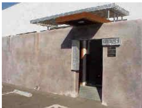
(Photo 4- Rear shop entrance)
