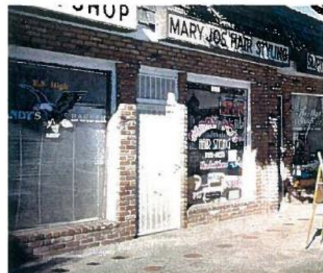
Photo 17 - Metal security door
