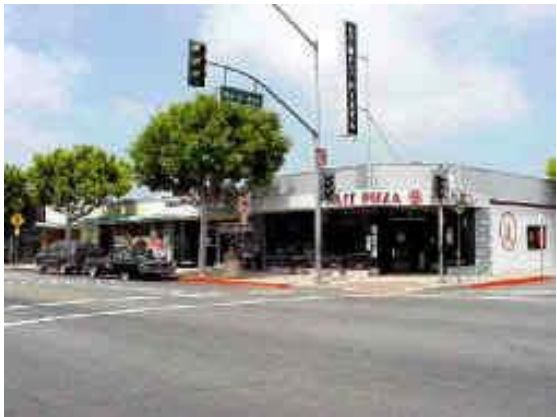
(Photo 3 – First floor constructed at Property line)
