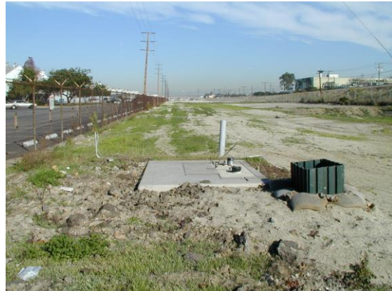
Figure 2: Northerly view of site.
