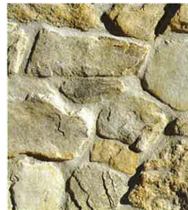
Grouted stone application example
