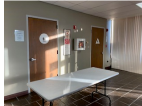
Figure 2 – Council Chambers lobby restrooms
