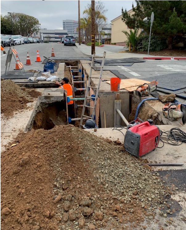
Connecting water lines at Indiana Street/Holly Avenue intersection
