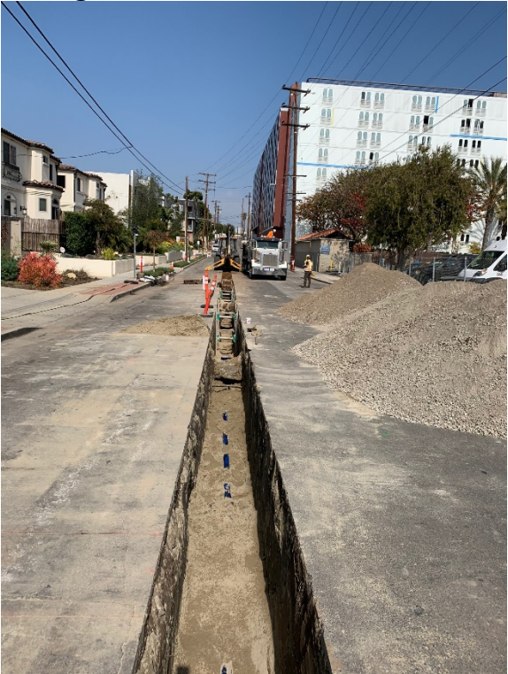
During: Installation of new water main on Indiana Street
