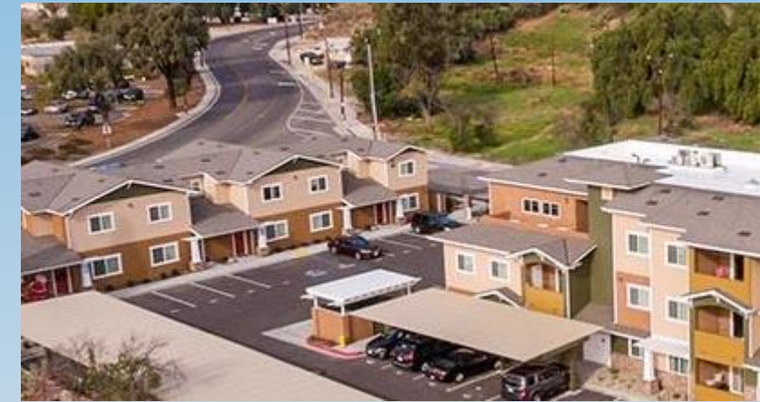
Walnut Street, 24 apartments, Moorpark
