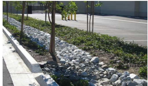
On-site storm water capture system
