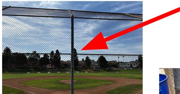
All cables or wires are attached to existing fencing and run to post and down to an outlet where the gamecam controller is located.
