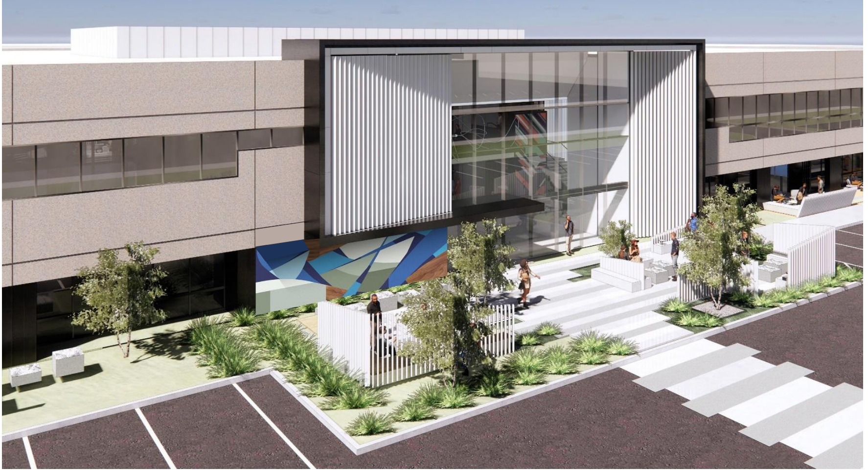
Mural: Pacific Blues (main lobby entrance facing Mariposa Avenue) Note: Rendering is for illustration purpose only. See page 8 for actual installation location.
