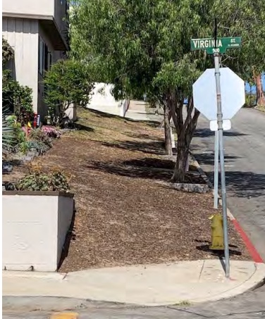
Before: 400 Block W. Mariposa Ave., looking west
