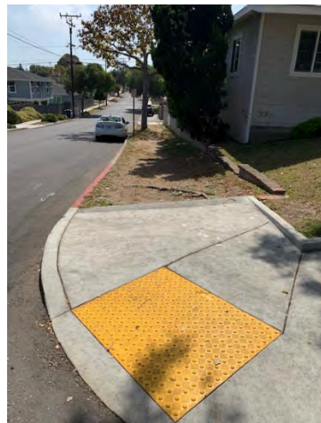
Before: 300 Block W. Pine Ave., looking east from Virginia St.
