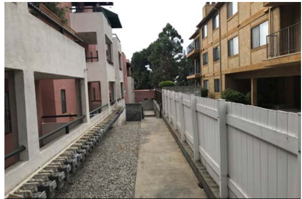
#10 NORTH PROPERTY LINE FENCE
