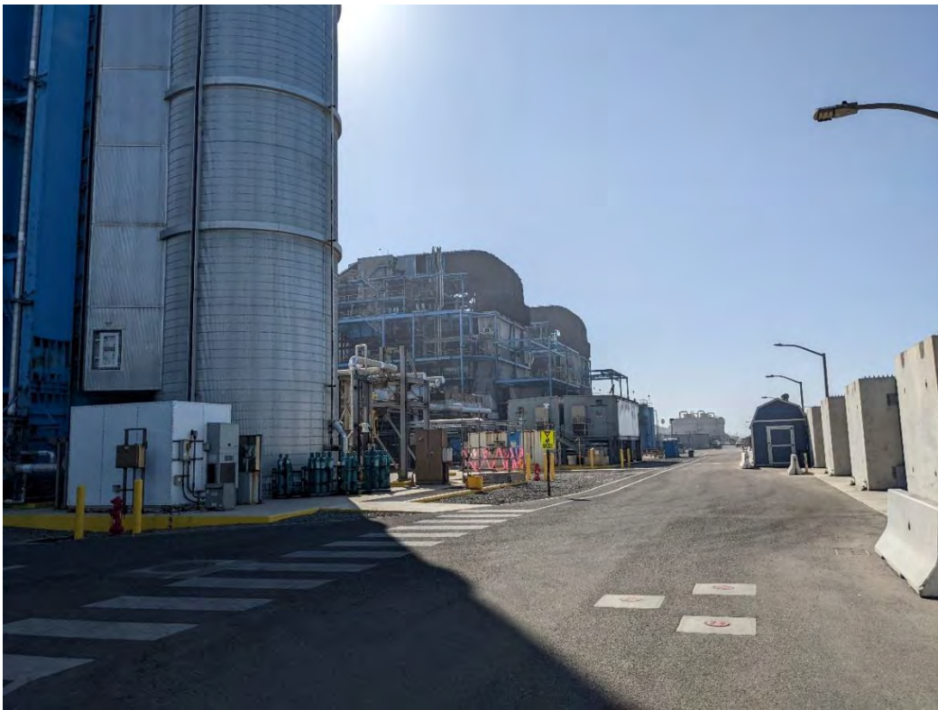
Photograph: 29 | West side of the NRG property facing south towards the project
