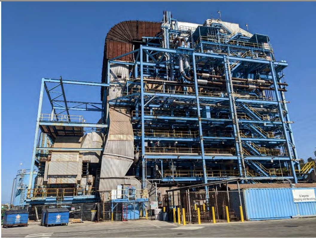
Photograph: 25 | Adjacent to Unit 4 facing North
