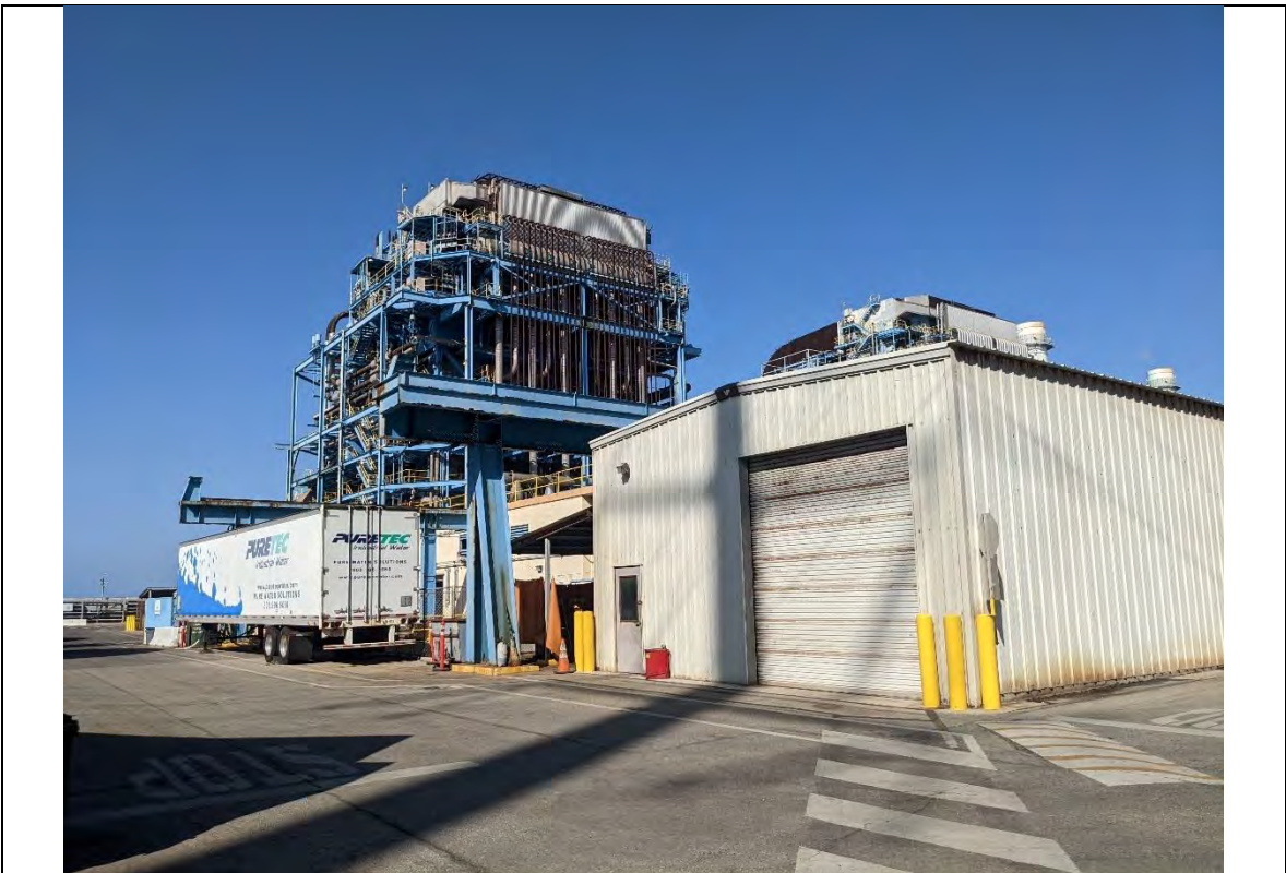
Photograph: 24 | Behind the South-East corner of Unit 4 facing West
