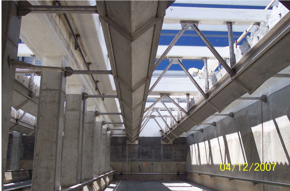
PRIMARY SEDIMENTATION TANK BAY
