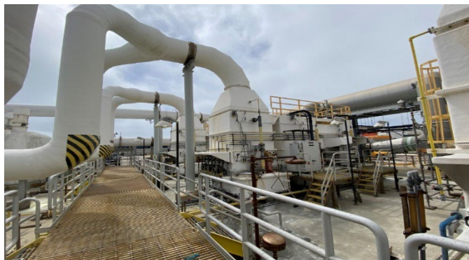
REFURBISH PRIMARY TREATMENT FOUL AIR SCRUBBERS
