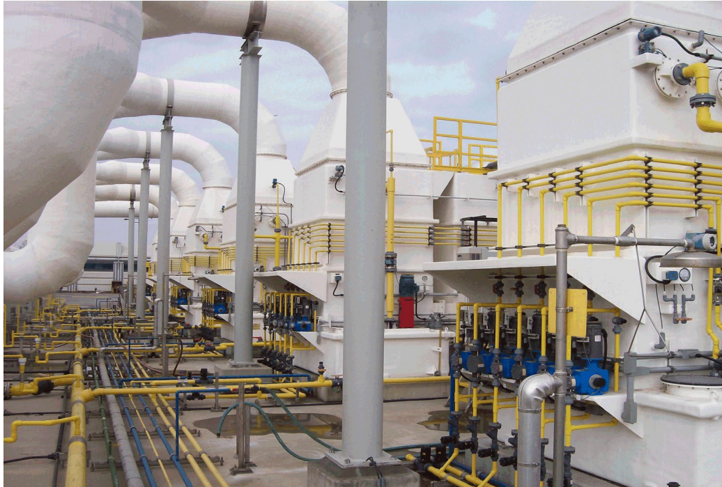
PRIMARY TREATMENT CENTRALIZED CHEMICAL SCRUBBERS
