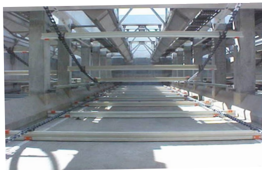
REPLACE SLUDGE HANDLING EQUIPMENT
