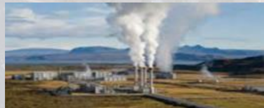
340 MW Geo, 14 MW Biomass
