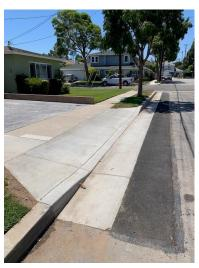
2. Before: Looking south on Loma Vista from W. Pine Ave. shows uplifted curb and asphalt. After: Looking north on Loma Vista toward W. Pine Ave. shows the problem tree was removed and new curb, sidewalk, and asphalt were constructed.
