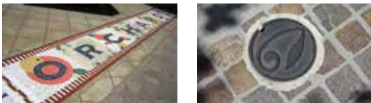
A variety of cohesive decorative paving materials creates vibrancy and identity for the Downtown
