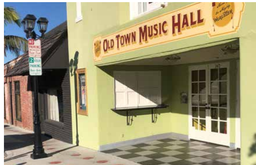
The Old Town Music Hall (140 W. Richmond Street) was built in 1921 and is a rare remaining example of a theater that was originally a live performance venue called the State Theater
