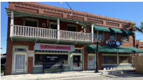
218-220 Richmond Street is one of the few remaining examples of a mixed-use commercial building from the 1910s
