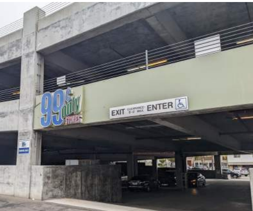
Entrance to the existing parking structure should be enhanced to more clearly depict a public parking garage
