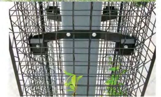
'GREENSCREEN' FITTED TO COLUMNS AND TARGETED BUILDING WALLS.
