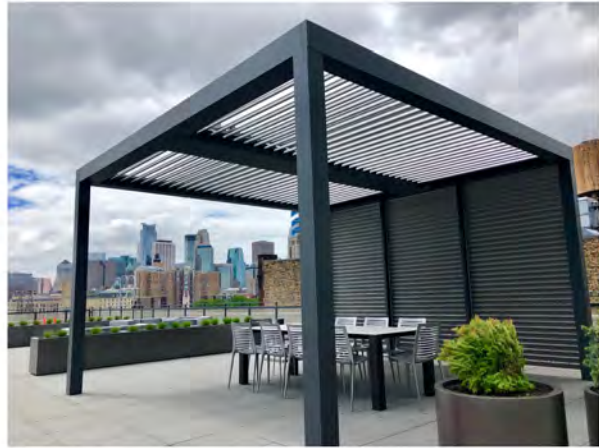
SHADE STRUCTURE WITH AUTOMATIC LOUVERS, LIGHTING, AND POWER GARAGE
